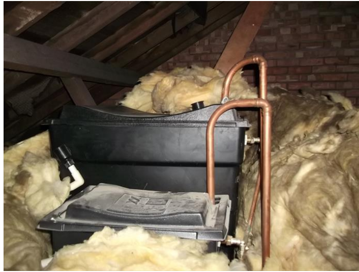
Title: Roof Space - Cold Water Storage Tank and F & E Tank
